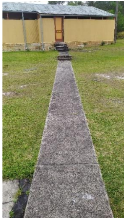
Concrete path behind P10 in good condition
