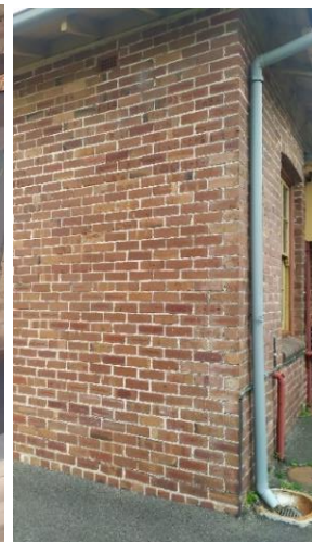
Brickwall with pointing in good condition P6
