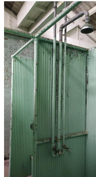
Above; inside A12 Showerblock
