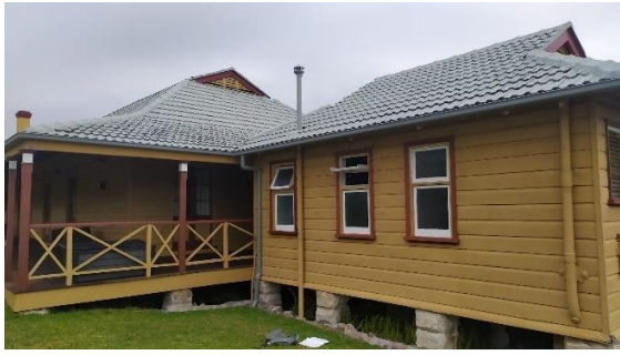
P9 demonstrating window functionality, roof and paintwork condition
