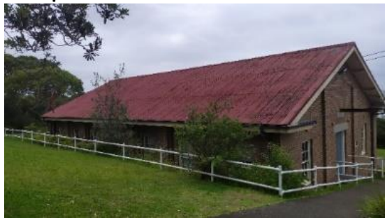
Fencing around A2 in good condition
