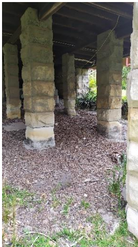
Sandstone pillars in good condition -P3
