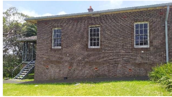
A20 Brickwork in good condition
