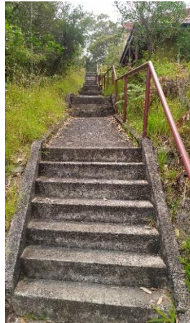
Concrete steps beside A25 in good condition
