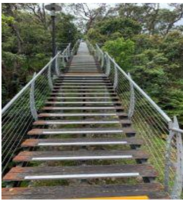
Nosing fixed to funicular stairs
